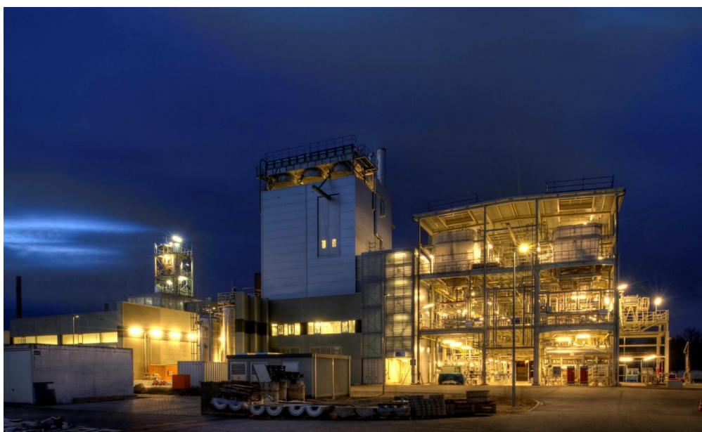
Figure 15: The bioliq pilot plant at the KIT in Karlsruhe, Germany, has a straw pyrolysis unit of 500 kg/h (2 MW) with bioslurry preparation, an high pressure, entrained flow gasifier with a capacity of 1 t/h bioslurry (5 MW) with hot gas cleaning and fuel synthesis unit operating at 55 bar. Copyright: Karlsruhe Institute of Technology
