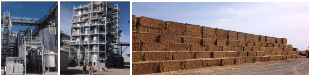
Fig. 4 Outlook of the LCB plant in Hugoton
